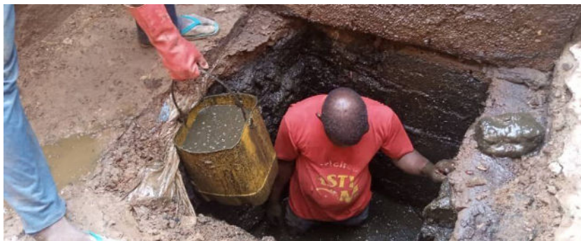
A bucket of sludge moves to the surface. Image Practica.
